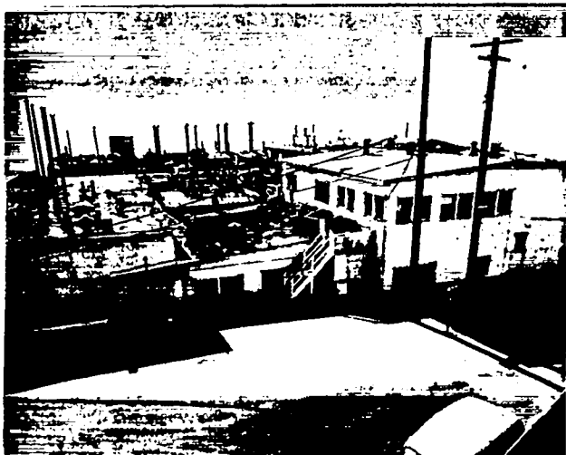
Fig. 1. The original wooden D Building which housed the chemists and metallurgists in CMR Division. Note that the chemical hoods of the laboratories on the first floor were vented individually, usually without filtration.
